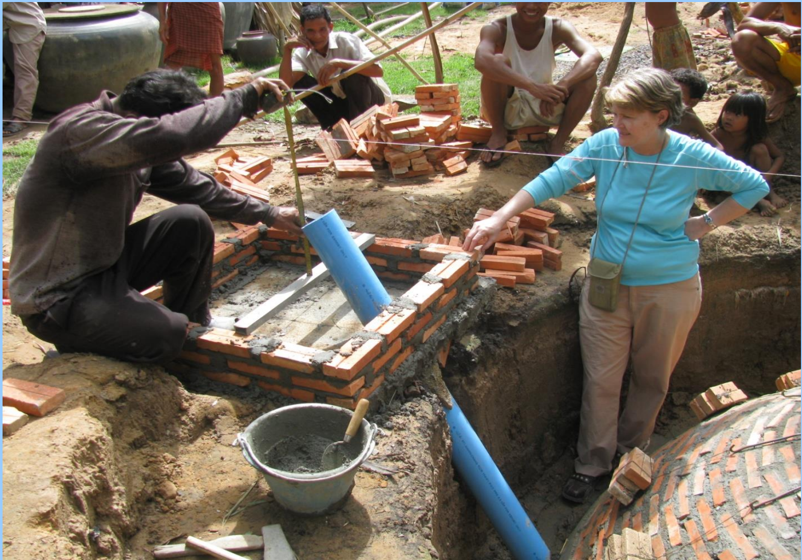
Biodigester under construction in Pursat, Cambodia – July 2010.
