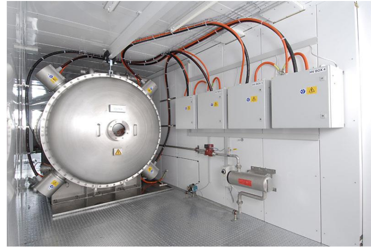
Ozone Generator (photo from Degremont)
